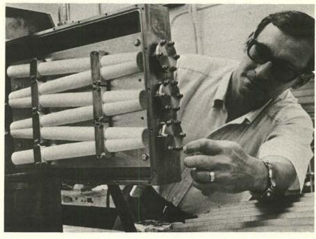
DAVE McARTHUR (5423) works on new laser which is excited by a fast burst reactor. Co-inventor is Phil Tollefsrud (5230A).
